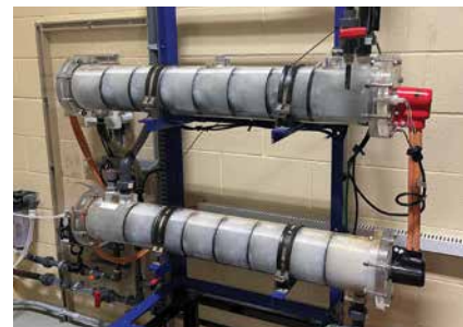
On-site sodium hypochlorite generation at Veolia's Columbia Water Treatment Plant.
