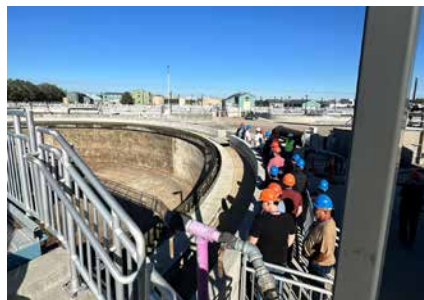
One half of our group touring a primary clarifier at WBWRF drained for maintenance.
