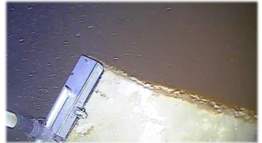
Finished Water Tank being vacuum cleaned – 1.5” Sediment
