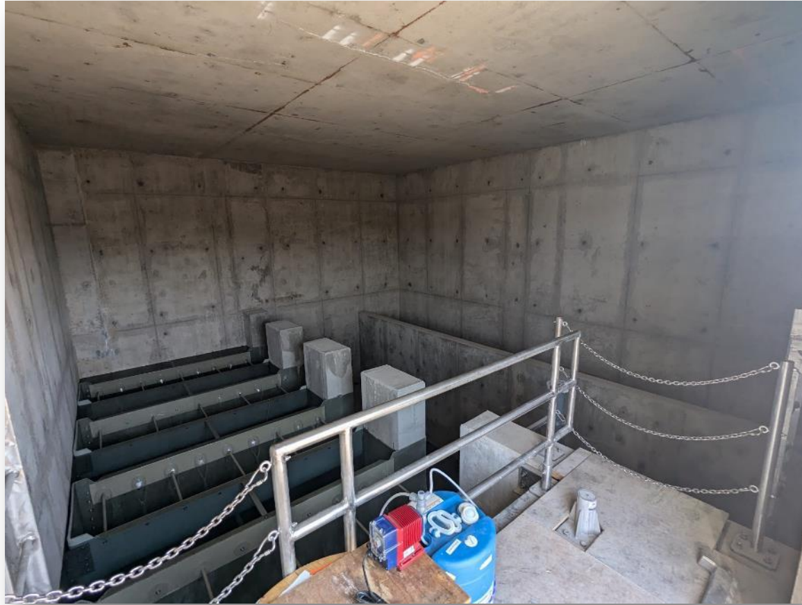
Dosing chemical at seal weir
