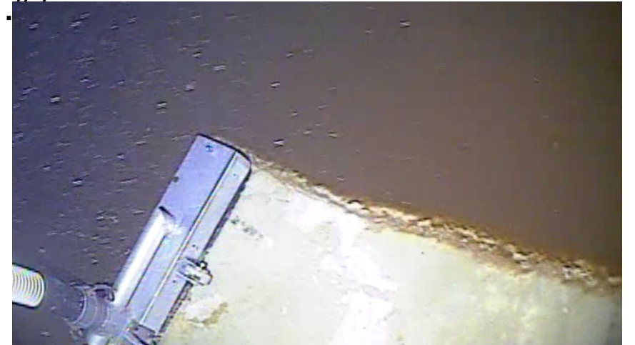
Finished Water Tank being vacuum cleaned – 1.5” Sediment
