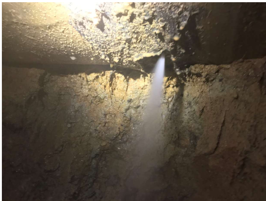
Pin-hole leak
