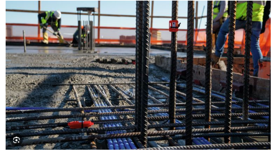
(In-Situ Strength & Temperature monitoring probes)
