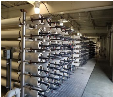
Membrane (Reverse Osmosis or Nanofiltration)
