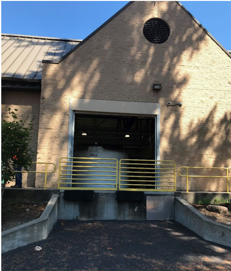
Front/South Side Overhead Door: 11'Wx10'H
