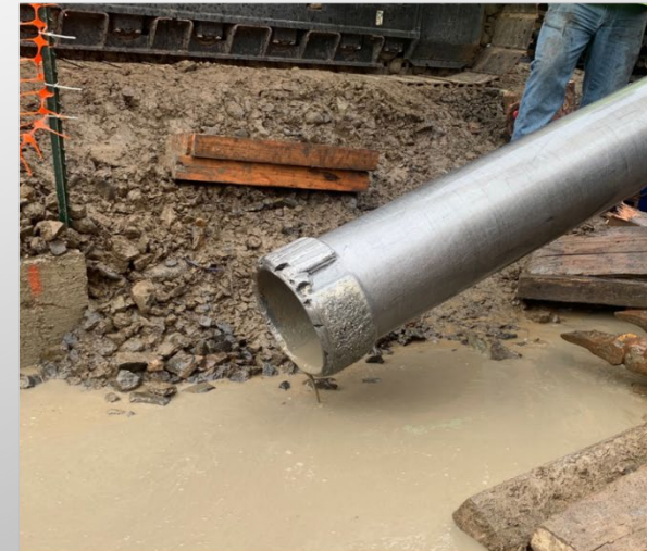
Cutting Shoe after 120 feet of Advance in the
