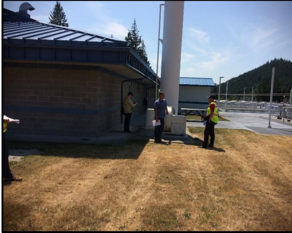
Figure 1-1. Existing Chlorine Scrubber and Layout Area for New Scrubber
