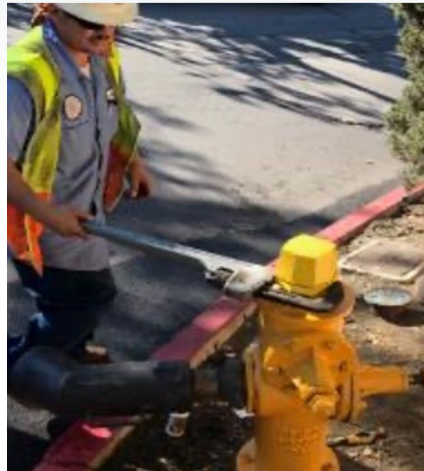
iHYDRANT® | INSTALLATION, LADWP
