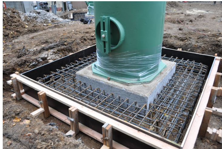
Expansion Foundation for Seismic Conditions
