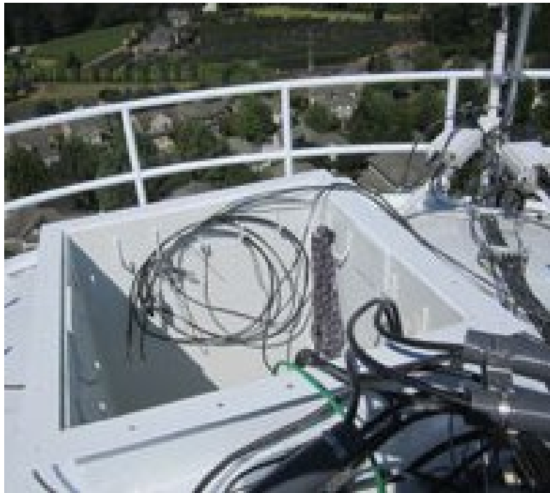
Dedicated Cell Cable Shaft at Top of Tank
