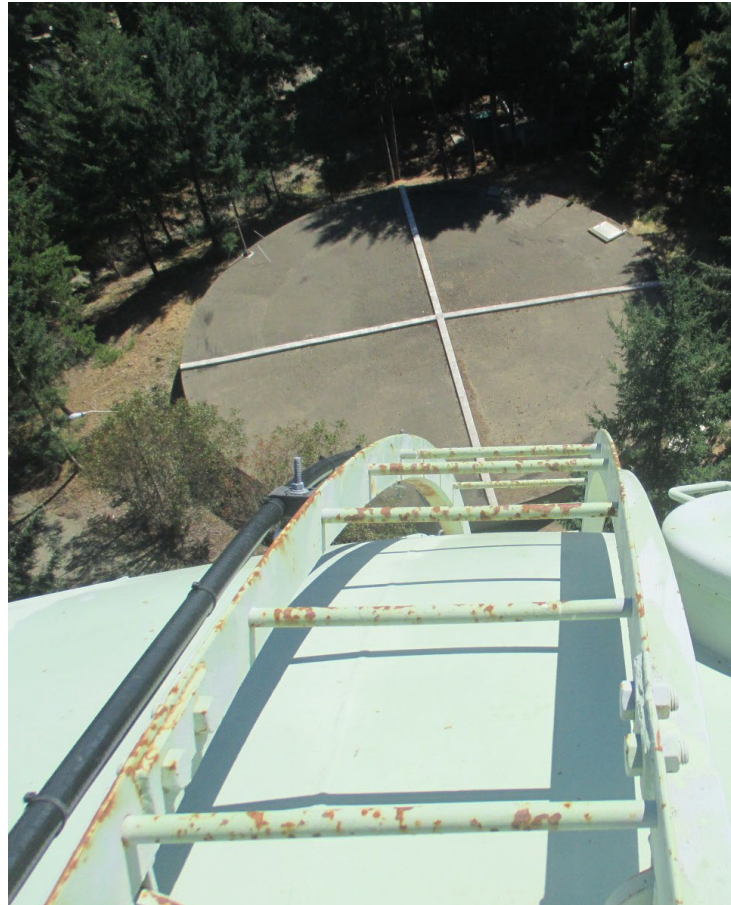
Challenging Roof Access
