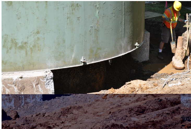
Replacing Foundation for Seismic Conditions
