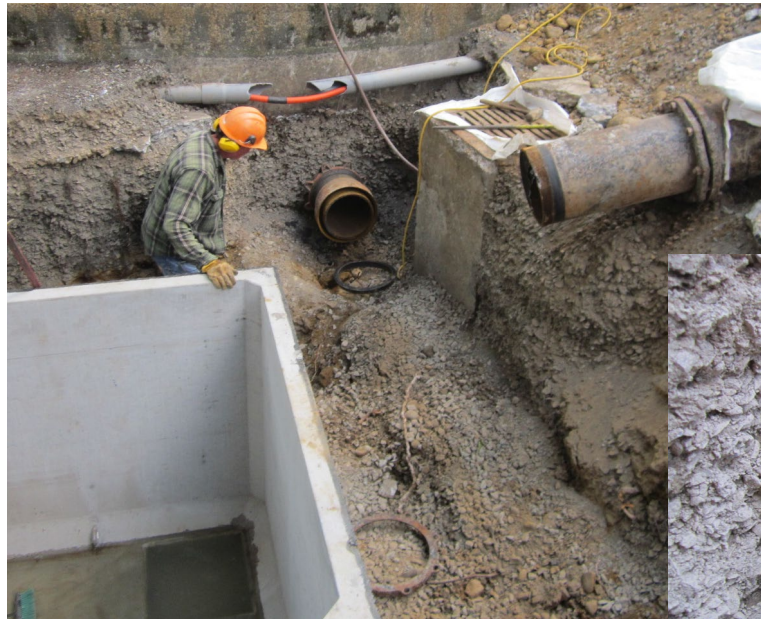
Existing Unrestrained Joint
