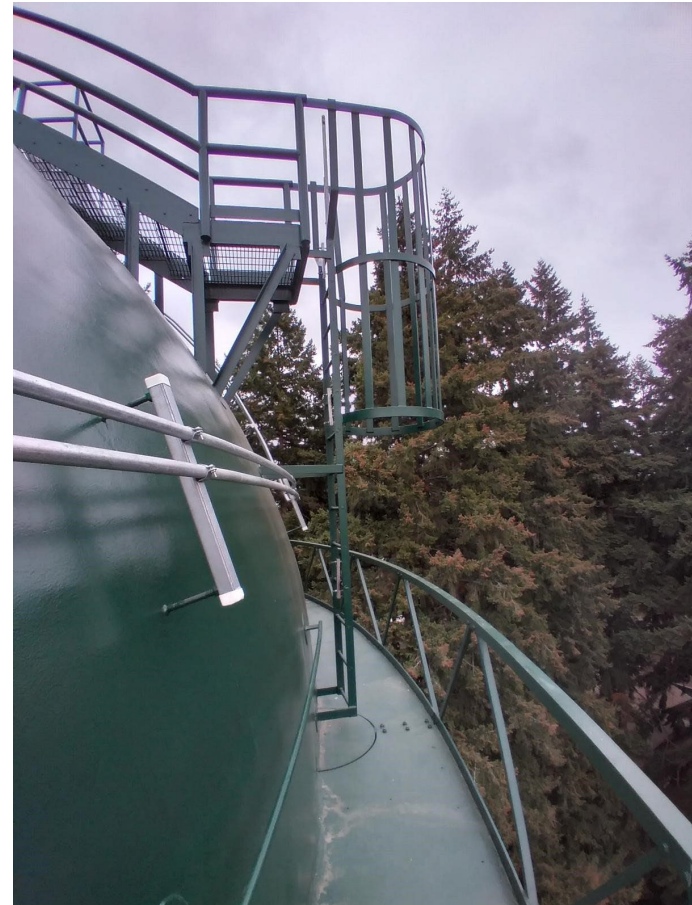
Improved Roof Access
