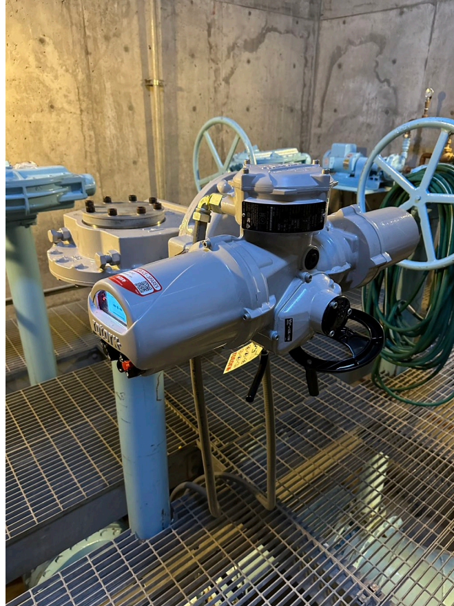
Electric Actuator Added to Existing BFV
