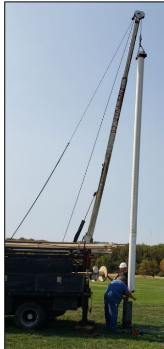
Liner/Screen Install
