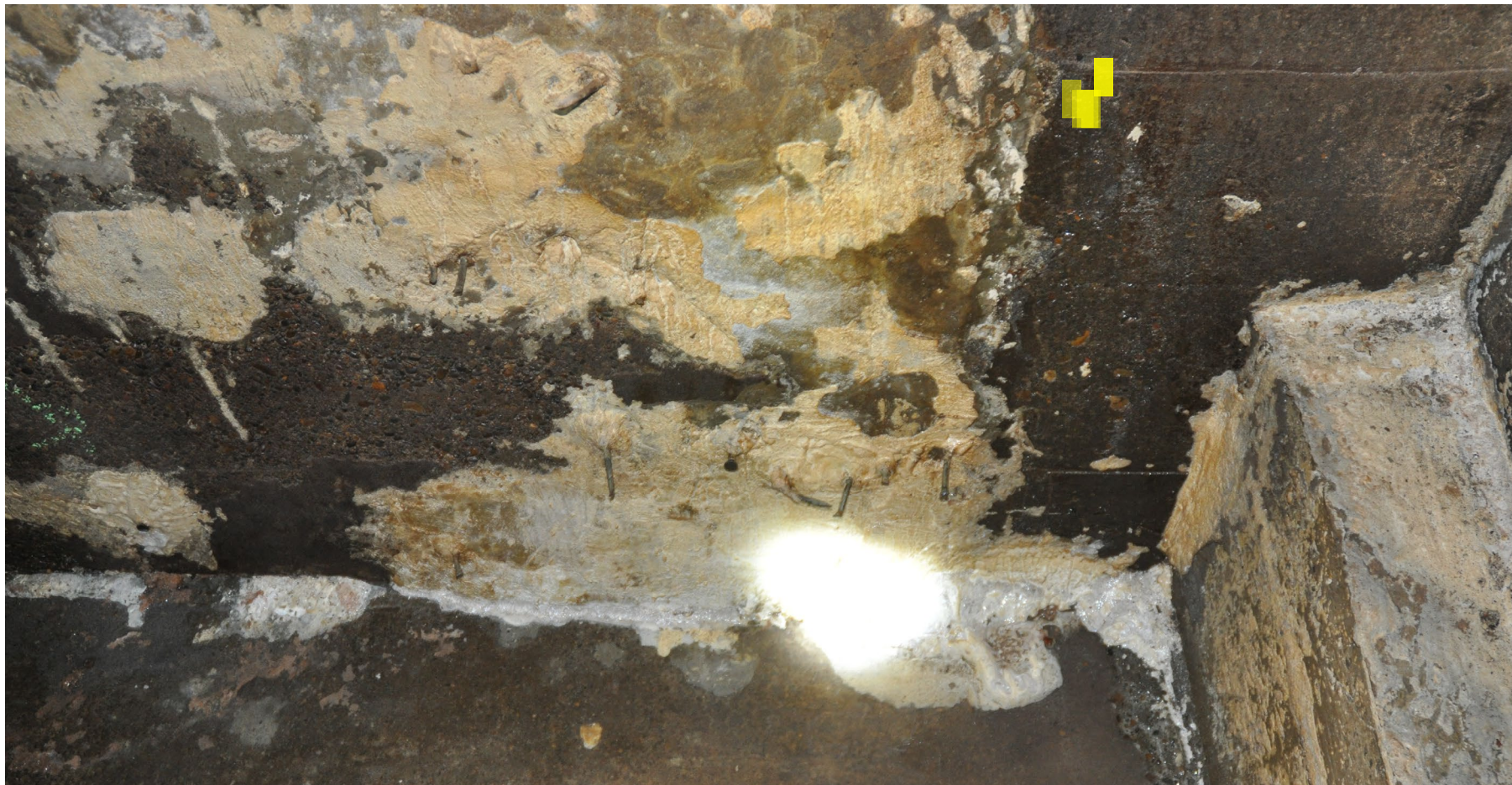
EAST WALL POLYURETHANE INJECTION
