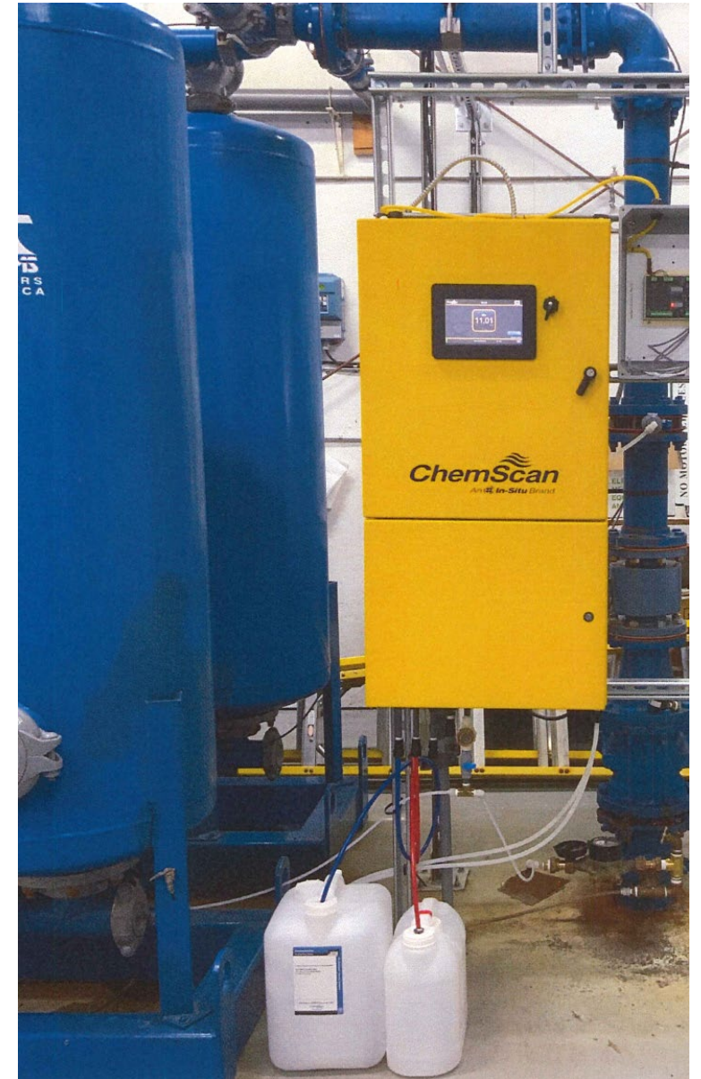
ChemScan NH 3 analyzer installed at end of 2021
