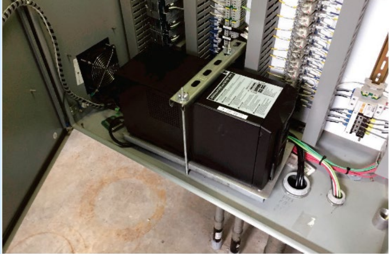
Figure 14 Battery in SCADA Cabinet
