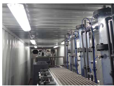
Filter and Floc/Sed Equipment inside enclosure.
