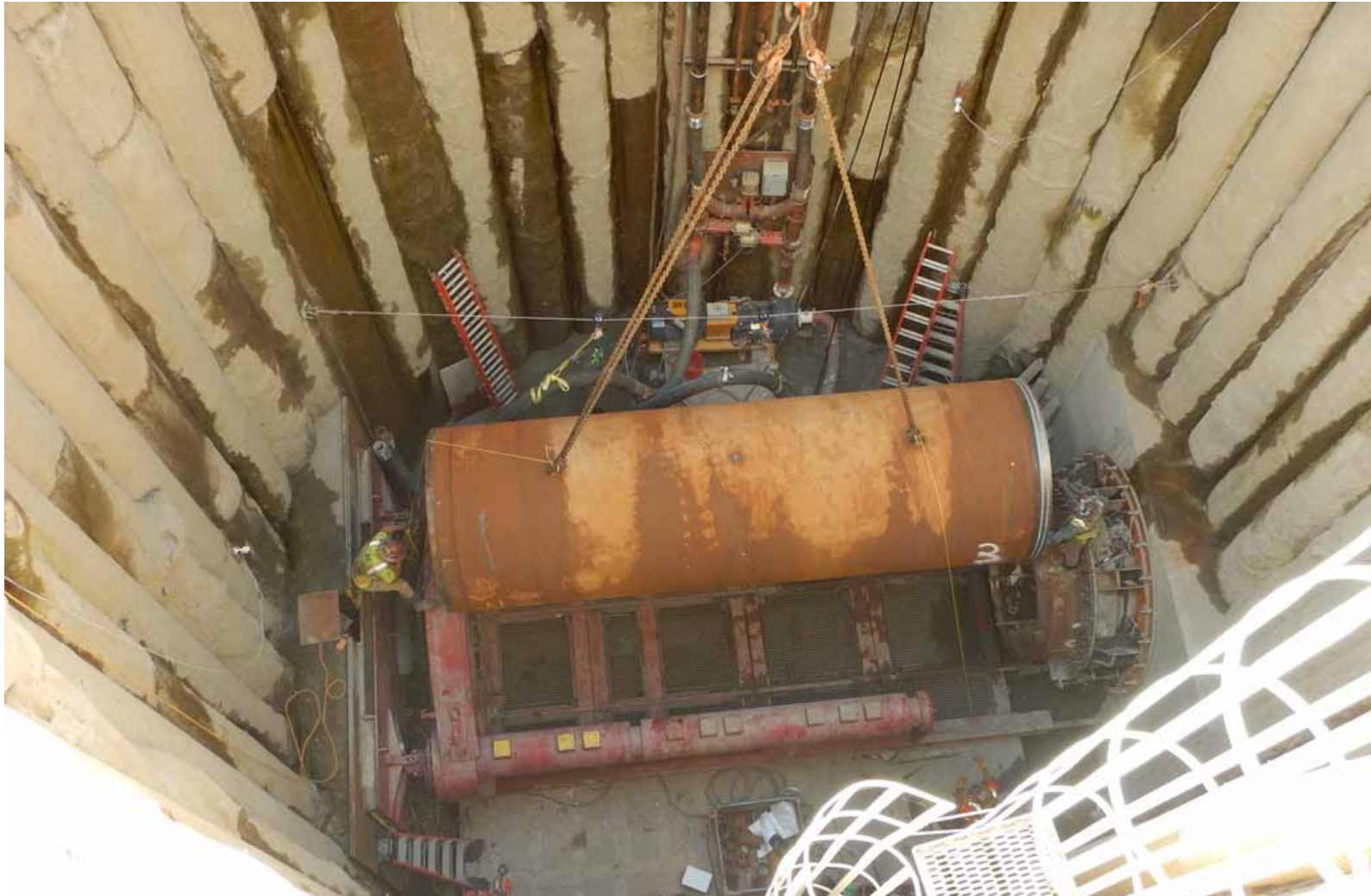
South Hillsboro Area Pipeline (PLW_1.3): Microtunnel of Butternut Creek, 84-inch casing pipe, setting next section
