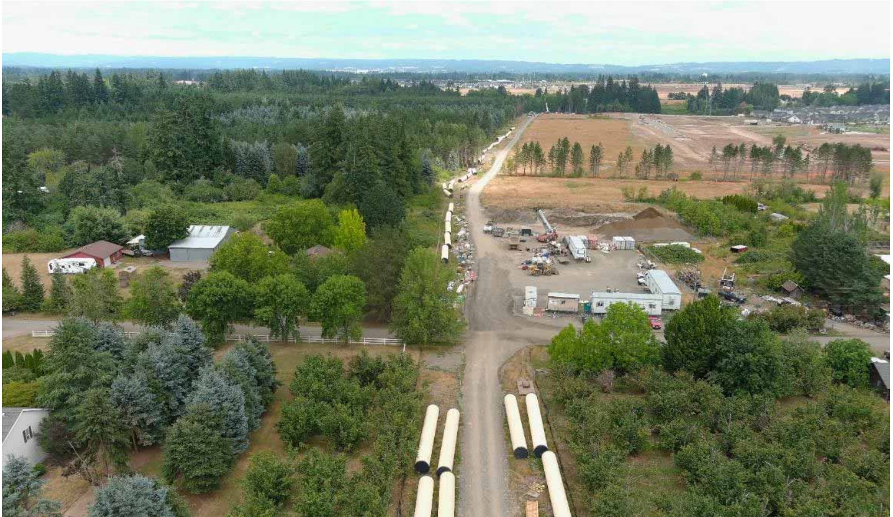
South Hillsboro Area Pipeline (PLW_1.3): Haul road and pipe laydown, staging area, creek crossing in distance
