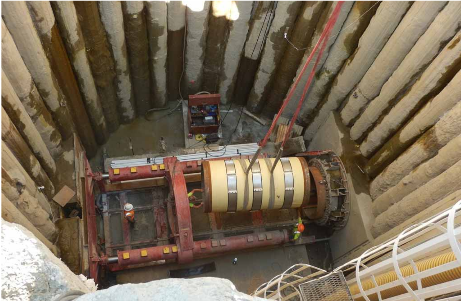
South Hillsboro Area Pipeline (PLW_1.3): Microtunnel of Butternut Creek, 84-inch casing pipe, 66-inch carrier pipe
