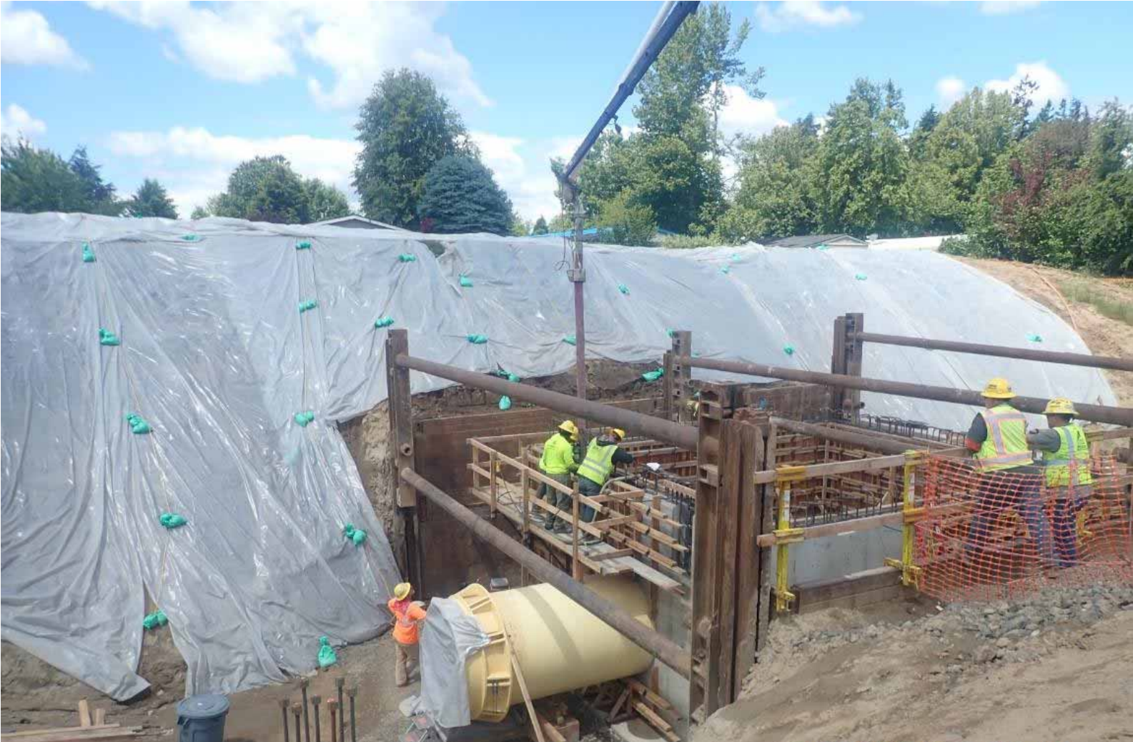
Raw Water Facilities Project (RWF_1.0) in Wilsonville: Placing concrete for flow meter vault walls 28 12:23
