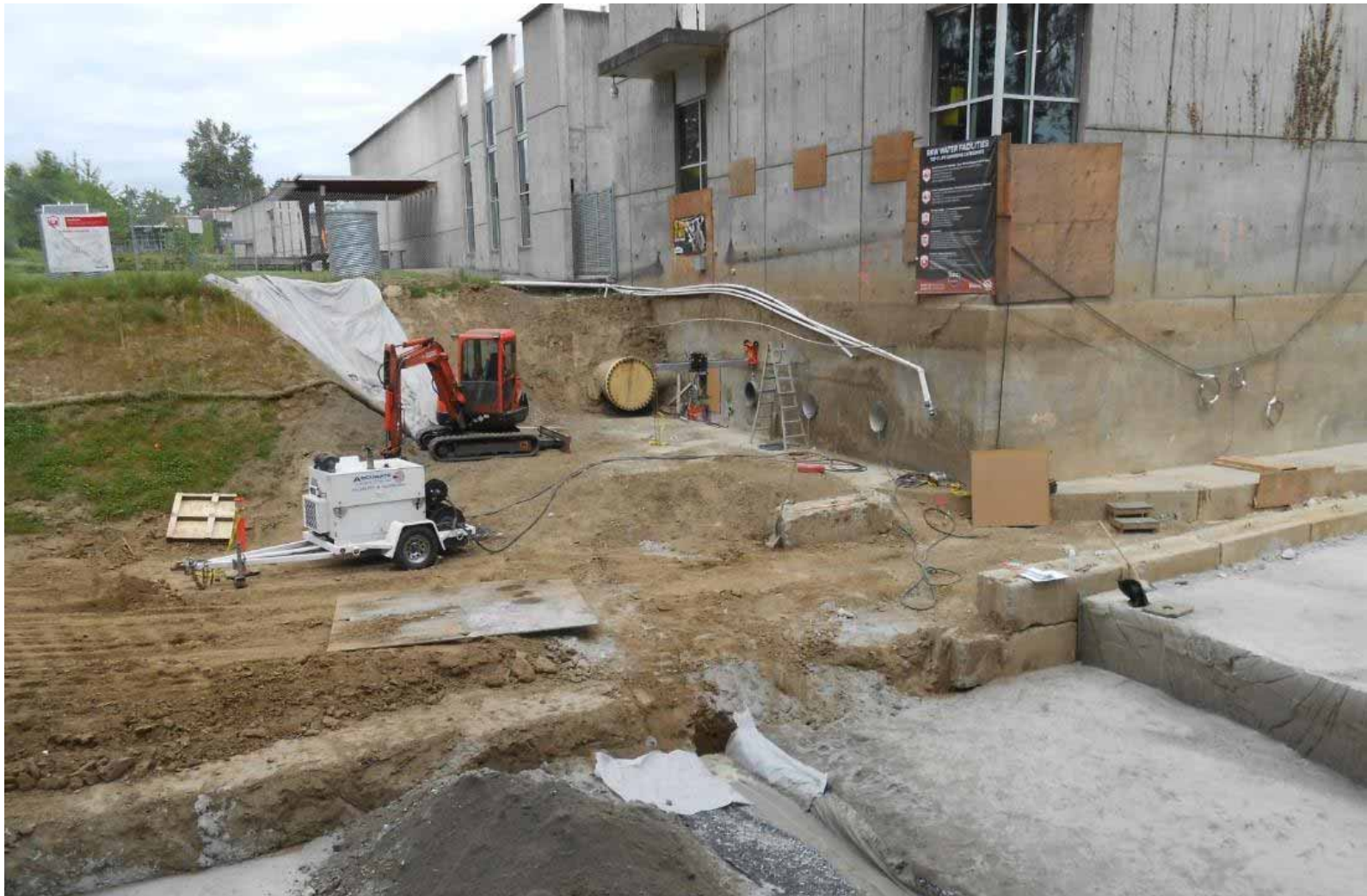
Raw Water Facilities Project (RWF_1.0) in Wilsonville: Preparing to install new pump header at raw water pump station
