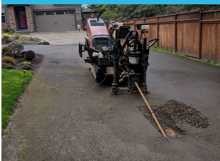
Bore Pit and tracer wire
