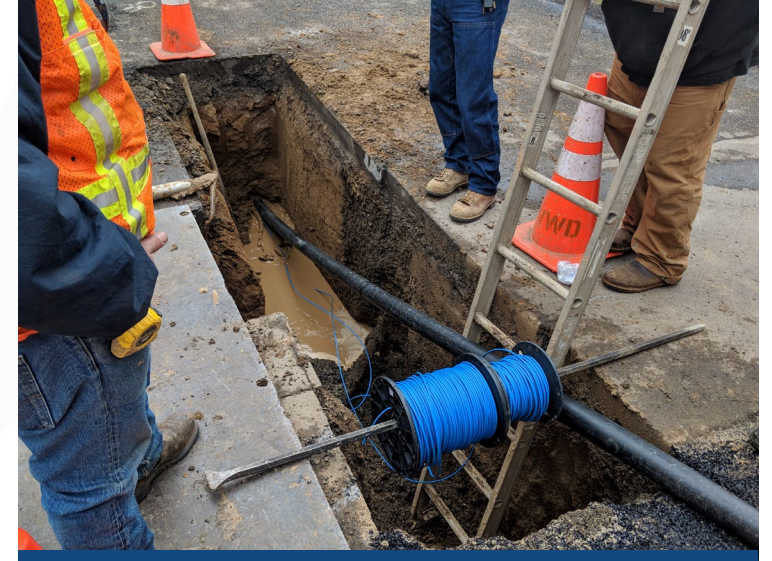
Bore Pit and tracer wire
