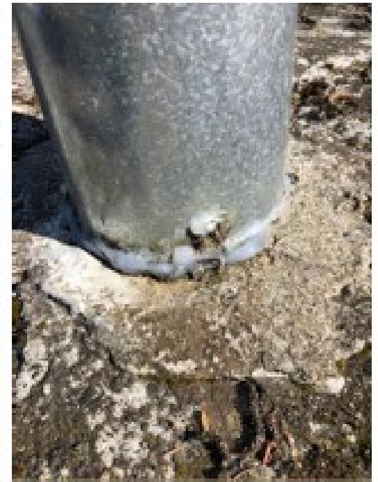
silicone seal on reservoir vent Poor
