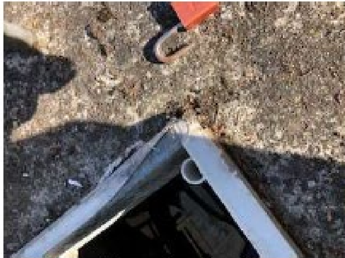
Weather strip seal on hatch – poor
