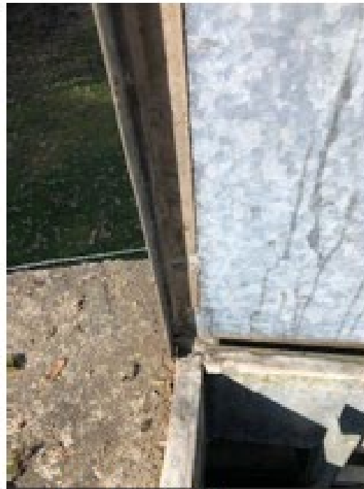
seal on hatch lid worn
