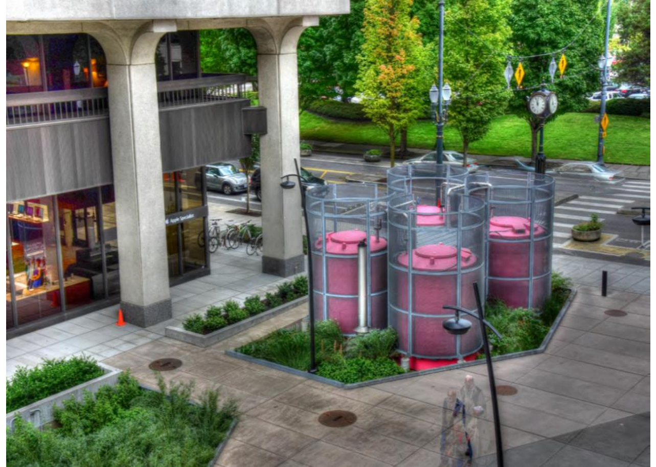
Natural Organic Recycling Machine (NORM) at Hassalo on Eighth, Portland, OR. Photo courtesy of Jim G. Maloney/Biohabitats, Inc
