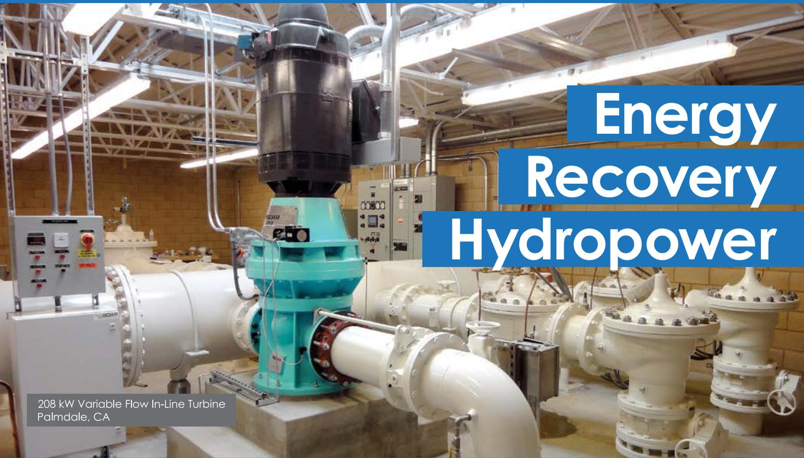
208 kW Variable Flow In-Line Turbine
