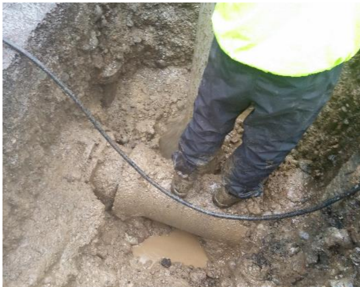
Leak Location (Before)
