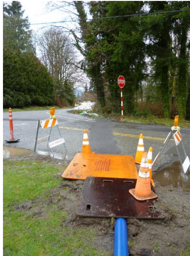
Crossing #2: Temporary Casing
