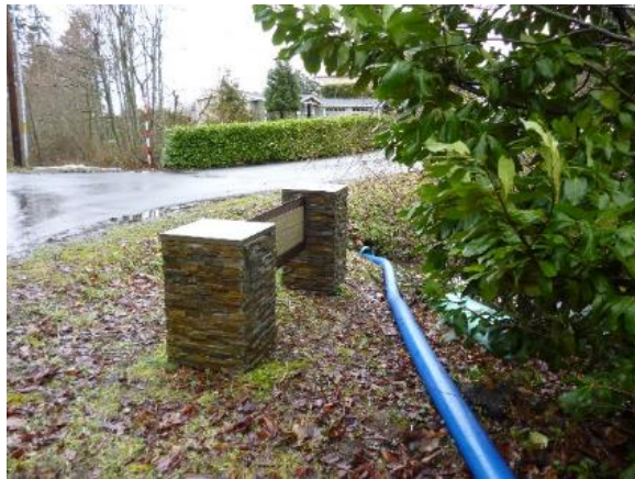
Crossing #1: Existing Culvert
