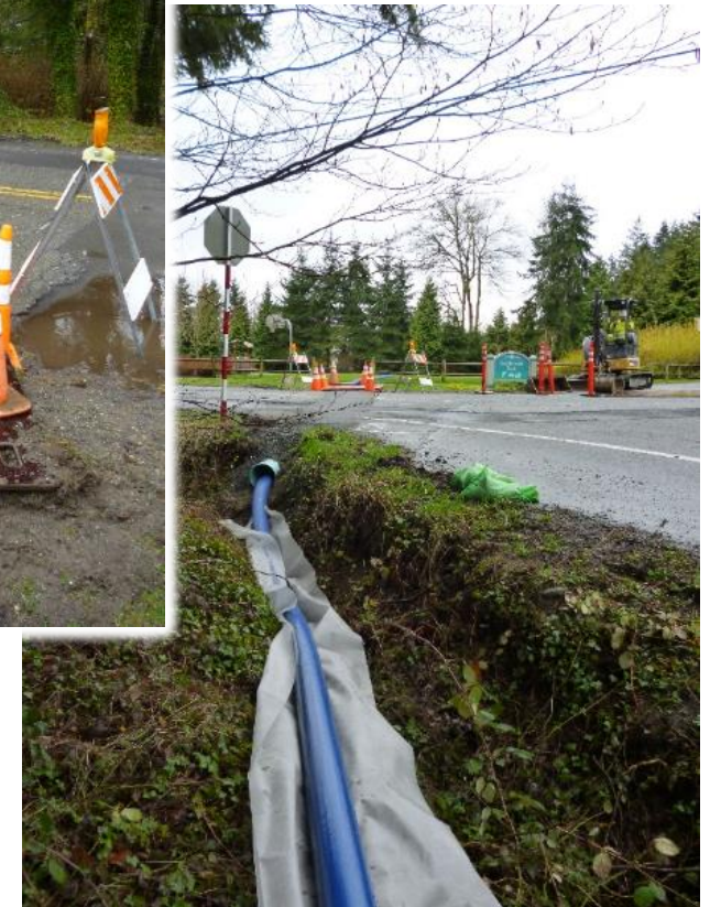
Crossing #2: Temporary Casing
