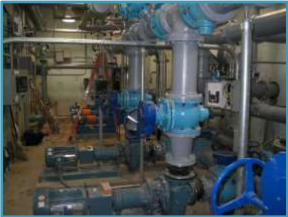
Filtrate Pumps in Background
