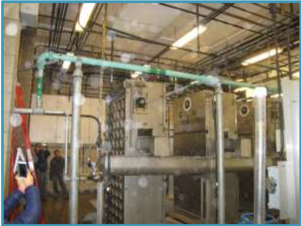
Band screens with 3- mm perforations
