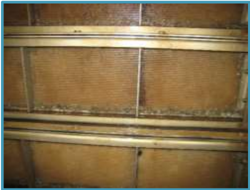
Band screens with 3- mm perforations
