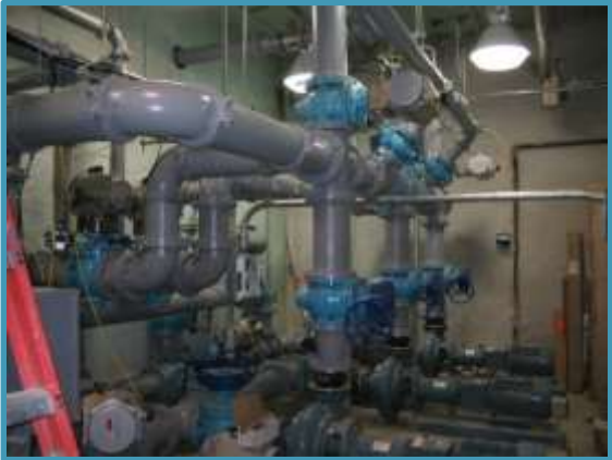
Membrane Recirculation Pumps
