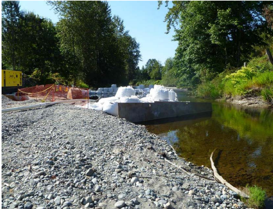
Viewing South, downstream. Sheets are set up against sandbag diversion.
