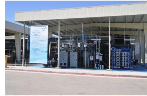
Source: City of San Diego Advanced Water Purification Facility
