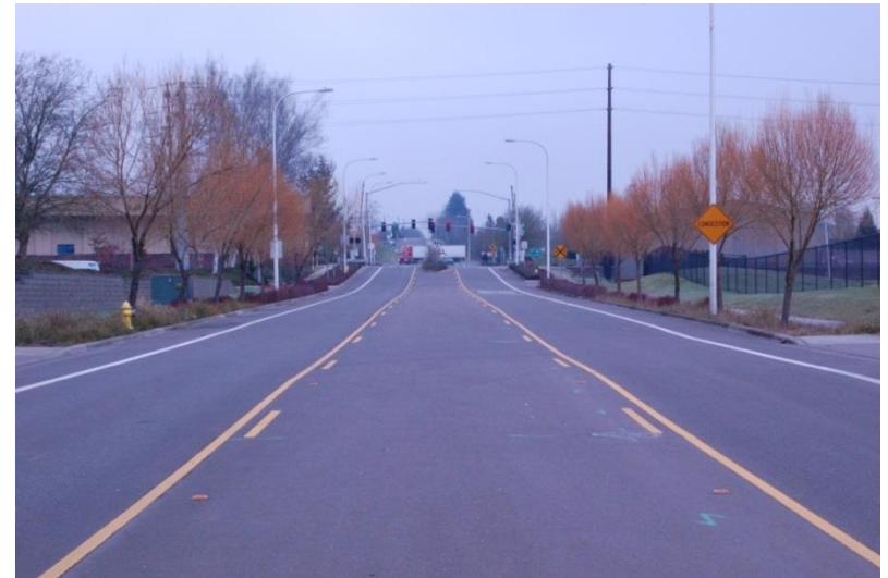
Boeckman Road in Wilsonville, looking east
