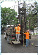
Crews conduct geological testing to determine soil conditions before pipe is installed.
