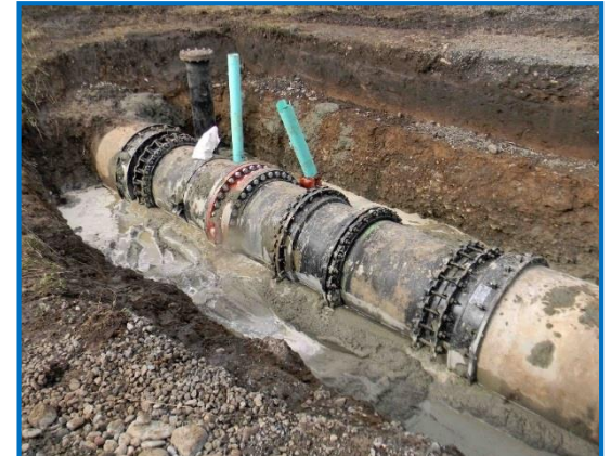
Cutting in 36-inch butterfly valves with custom fabricated transition couplings
