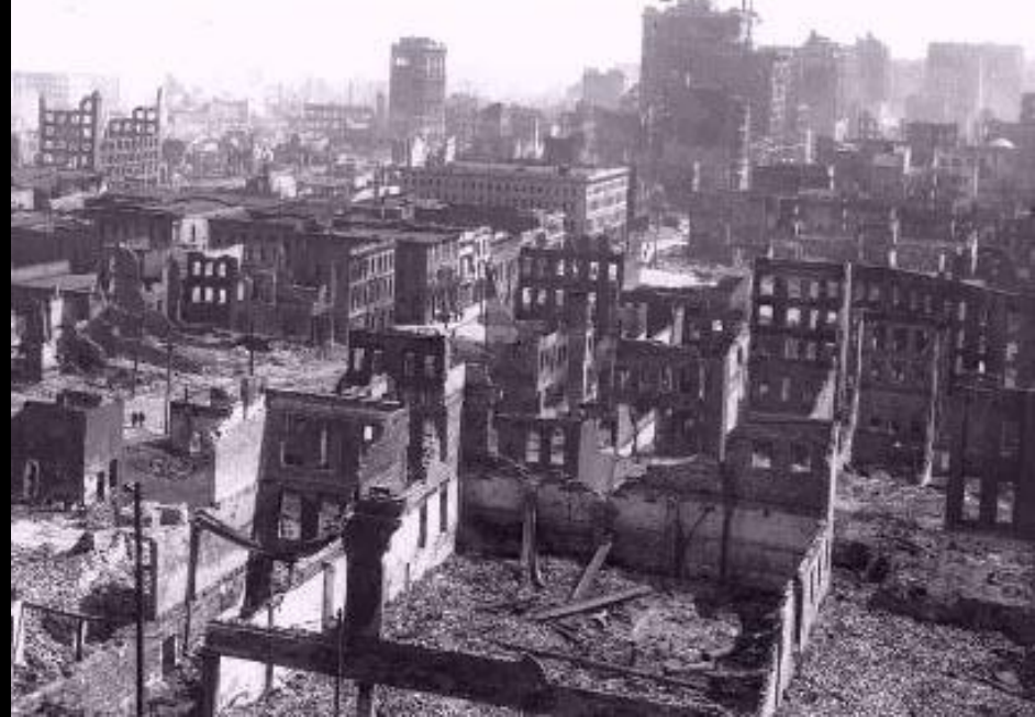
1906 San Francisco Earthquake
