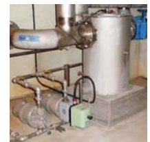
Sediment Trap with Electrically Actuated and Manual Drip Traps
