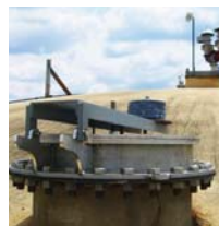
Emergency Vent and Pressure/Vacuum Vent and Flame Arrester
