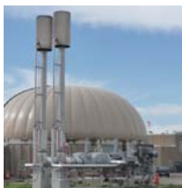
Ground Level Pilot Waste Gas System
