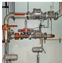
Regulator and Flame Trap Assembly
