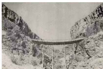
Timber Trestle Supporting Wooden Flume
