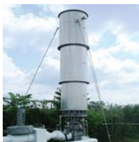
Enclosed Waste Gas Burner
