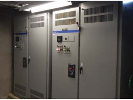
VFDs for the pump motors at the new intake
