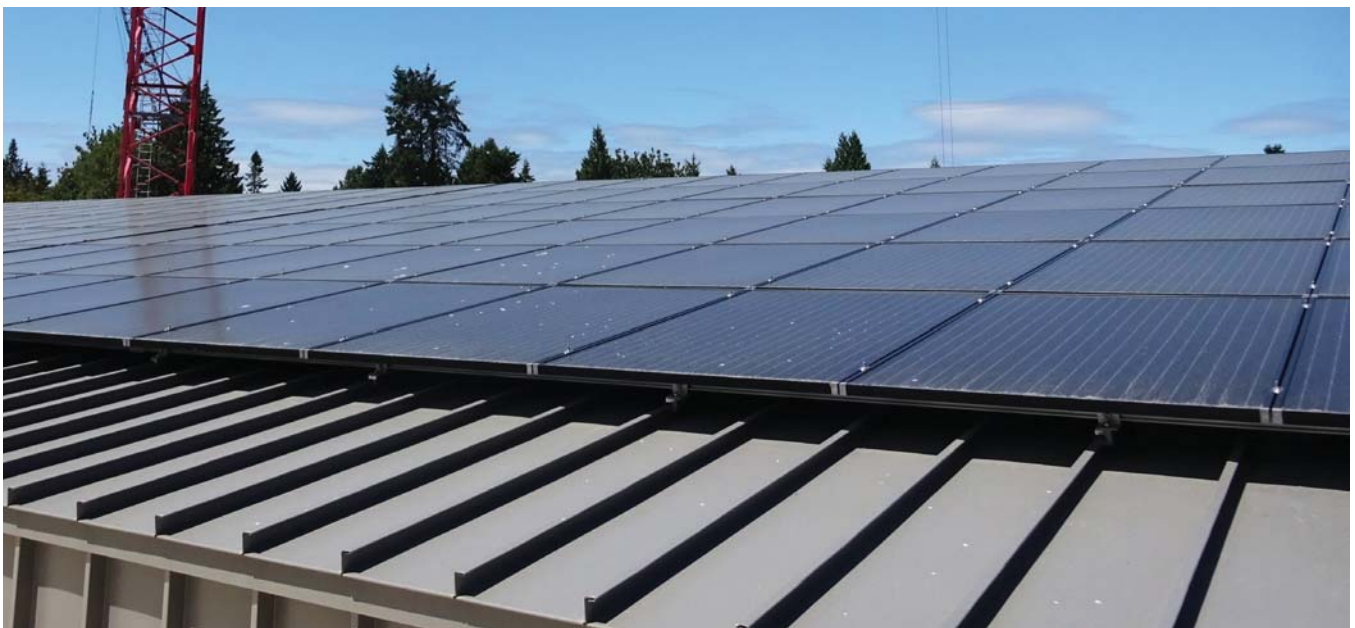
Solar panel array on the electrical building at the new water treatment plant
