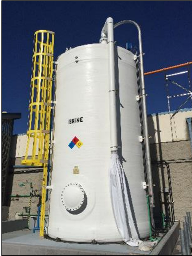
Brine Tank 4m Diameter
