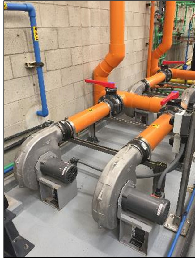
Hydrogen Dilution Blowers
