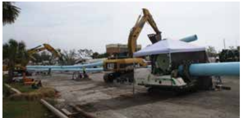
Two pipe strings are arranged in position to complete first Intermediate fusion joint.
