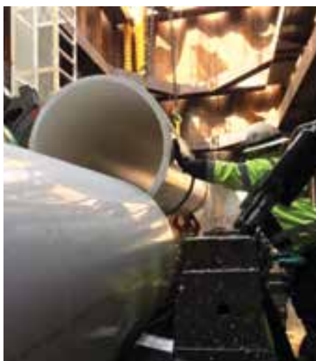
Pipe being lowered into pit to prepare for fusion.
