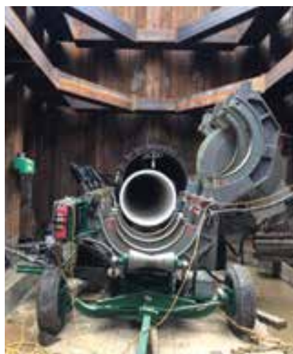
Fusion machine and pipe setup inside pit.
