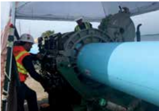
Fusion technician completes new fused joint on pipe.
