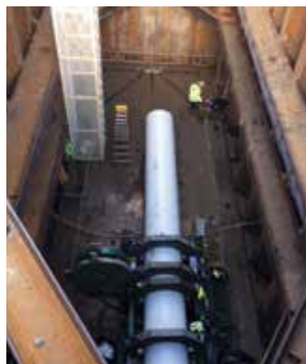
In-pit fusion of pipe.
