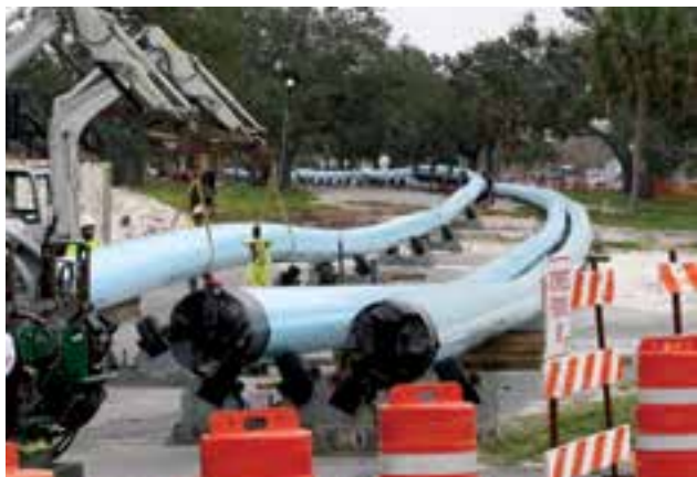
Pipe staged side-by-side for intermediate fusion.
