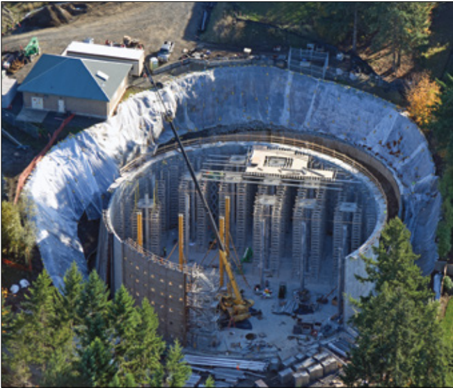
The new Grabhorn Reservoir was offset from the old reservoir's position so the old walls could be used as shoring.
