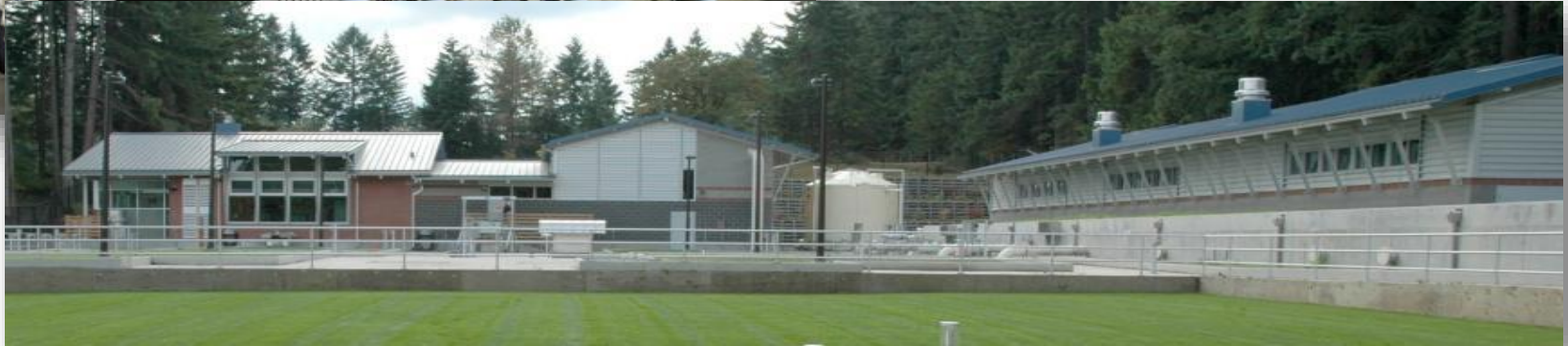
Martin Way Satellite Reclaimed Water Plant
