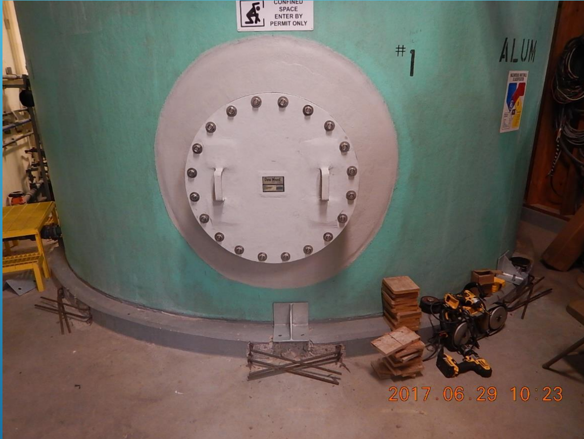
Seismic life safety improvements – equipment bracing
