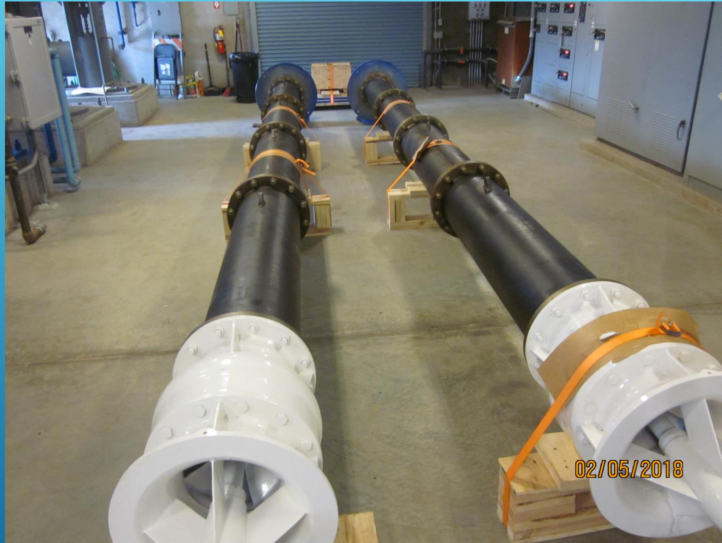
Backwash pump replacement in kind
