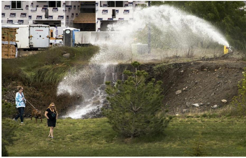
Airway Heights Public Work Department flushes potentially contaminated water from a fire hydrant into Aspen Grove Park in Airway Heights, Friday May 19, 2017. The city is working to remove contaminants from the water pipes caused when chemicals used for fire suppression at Fairchild Air Force Base entered the water supply. (Colin Mulvany / The Spokesman-Review)
