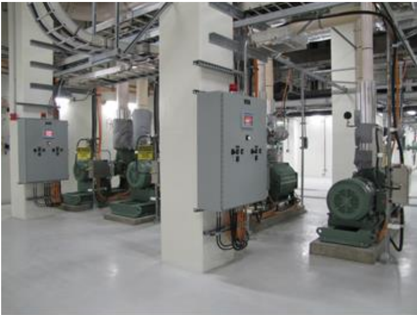
Grit distribution channel and grit tank blowers
