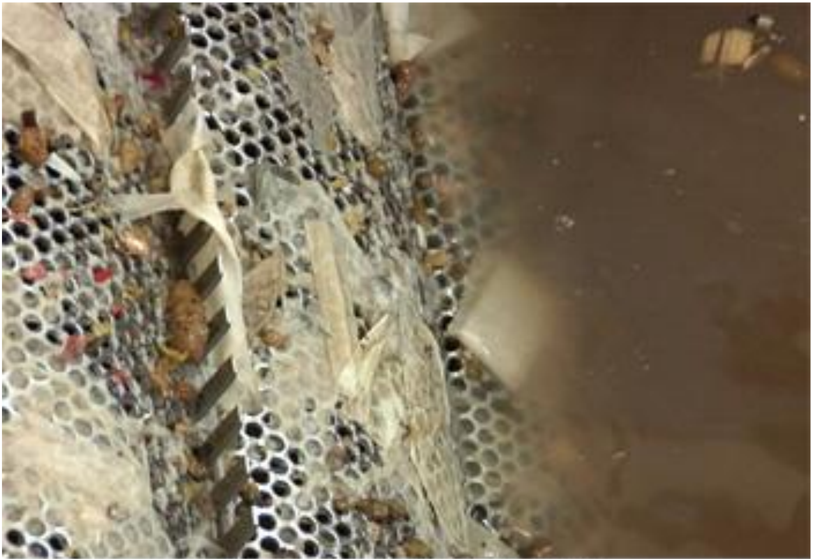
Debris captured by the screen panels
