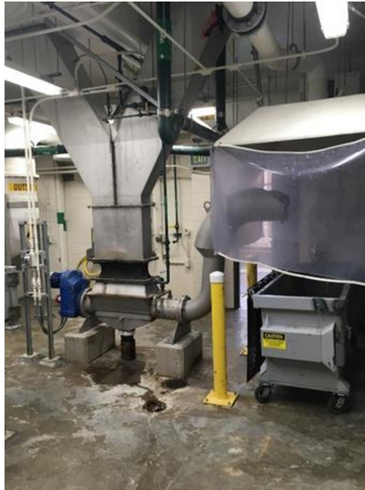
Screenings grinder compactor
