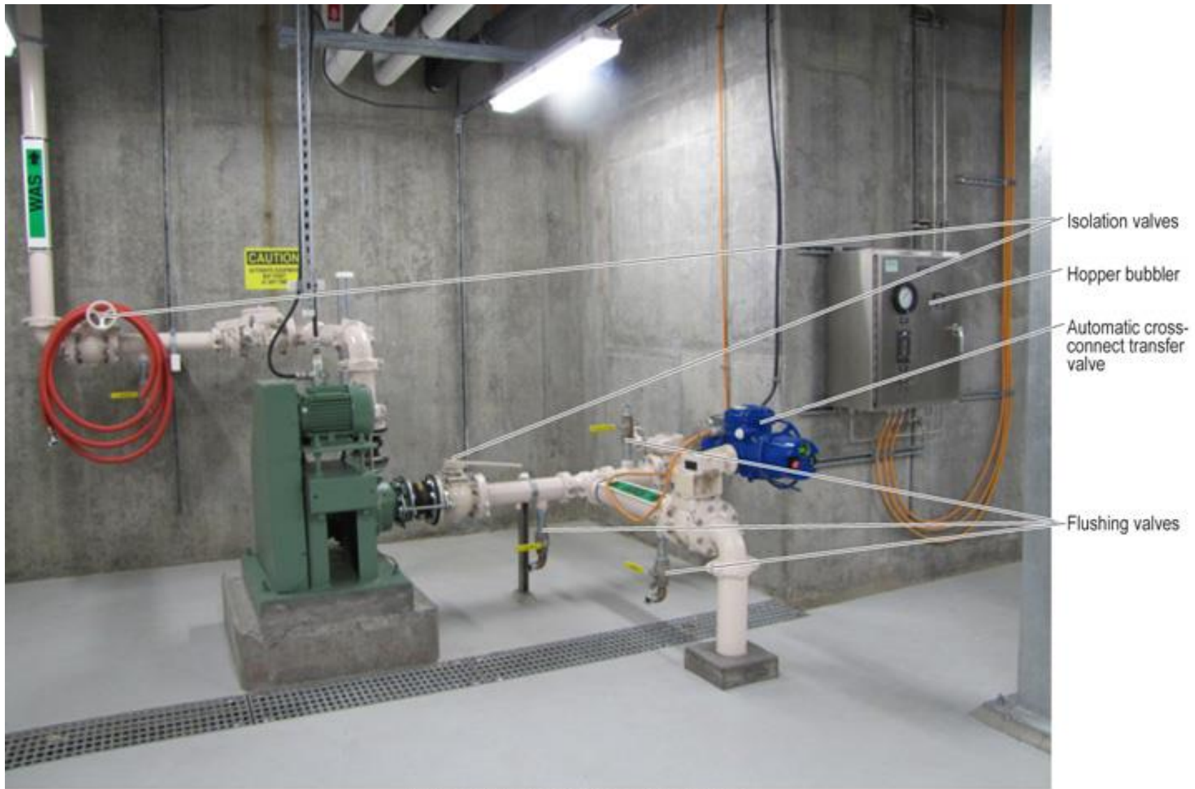
Primary effluent screenings hopper pumps
