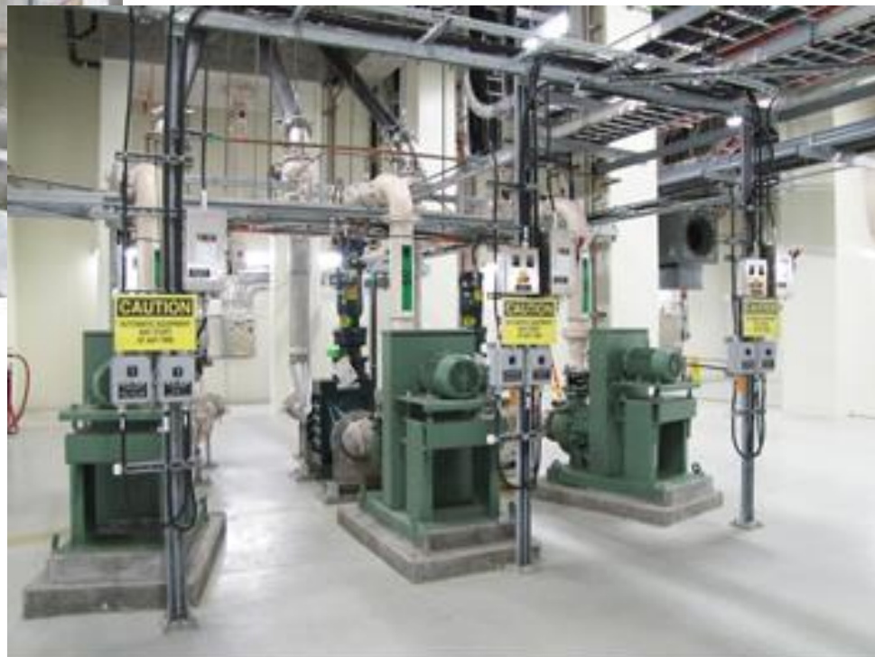
Influent screenings sump grinders and pumps
