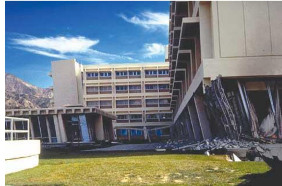
Severe damage to the Olive View Hospital in San Fernando, California due to the 1971 San Fernando Earthquake (Source: USGS)
