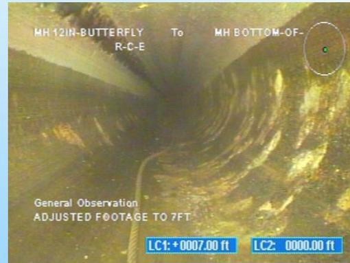
Six Gushers – Point repairs not done but no gushers this time around. However, City decides to move forward with point repairs prior to lining.
