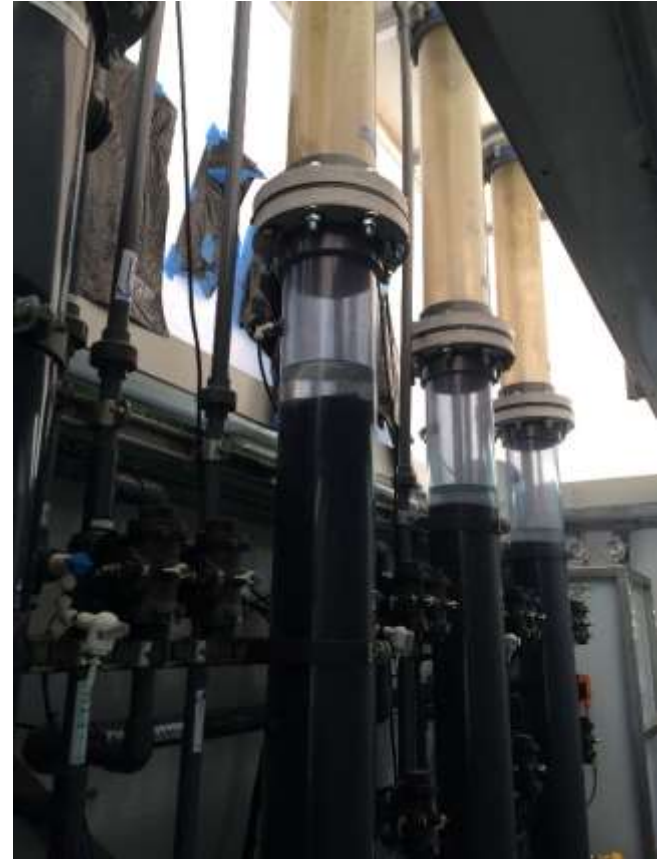
Pilot Plant Filters
