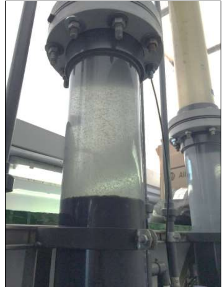
Filter backwashing in progress
