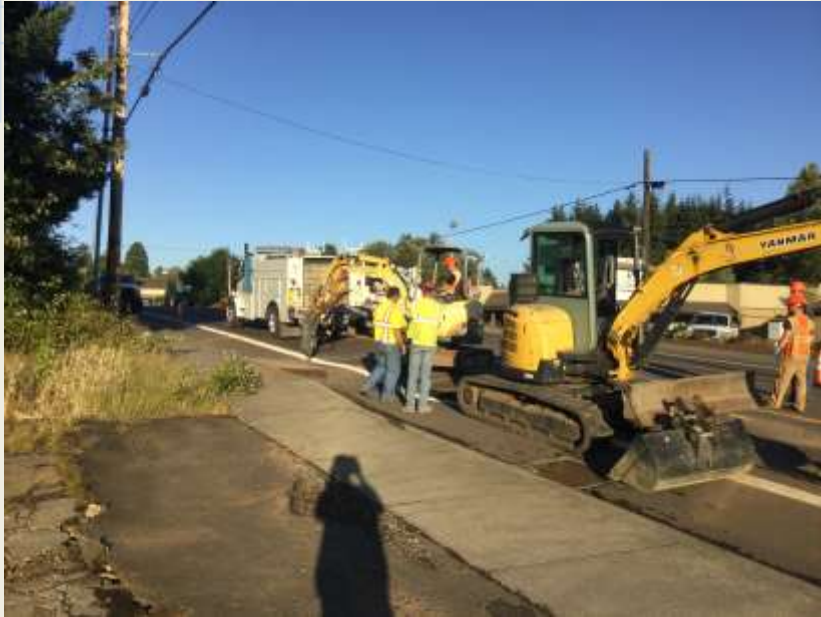
Repair broken pipe: On-call Contractor
