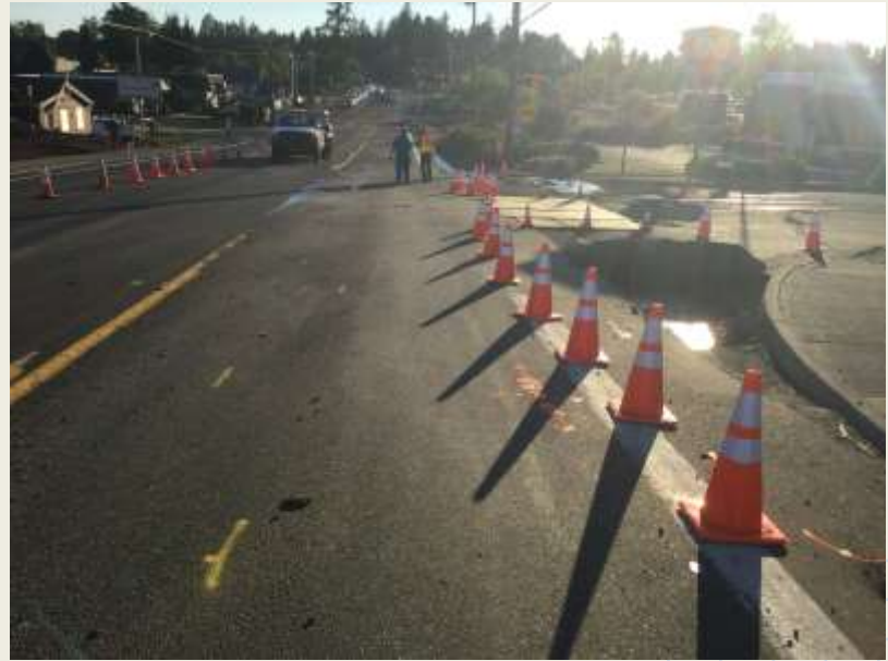
Restore Access (Release Trapped Cars)
