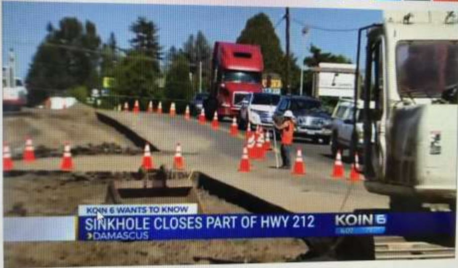
KOIN 6 News Staff - DAMASCUS, Ore. (KOIN) — About 1,500 water accounts with Sunrise Water Authority were under a boil water notice because of a water main break in Damascus.
