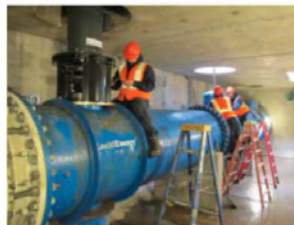
Lucid Energy installed four electric generators inside a Portland drinking water pipeline.
