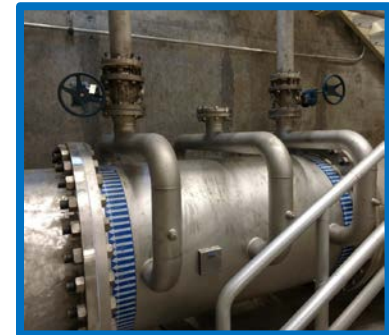
Ozone injection equipment at the Lake Oswego – Tigard WTP
