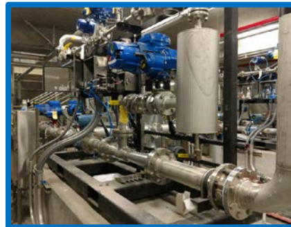
Ozone injection equipment at the Lake Oswego – Tigard WTP
