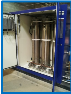
Ozone generation equipment at the Willamette River WTP, Wilsonville
