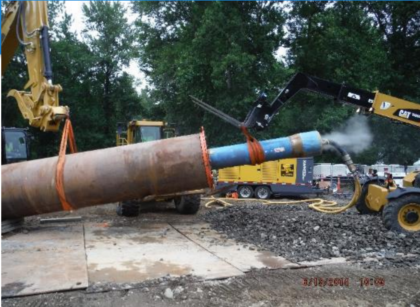
Pipe Ramming Used to Install 60-inch Conductor Casing
