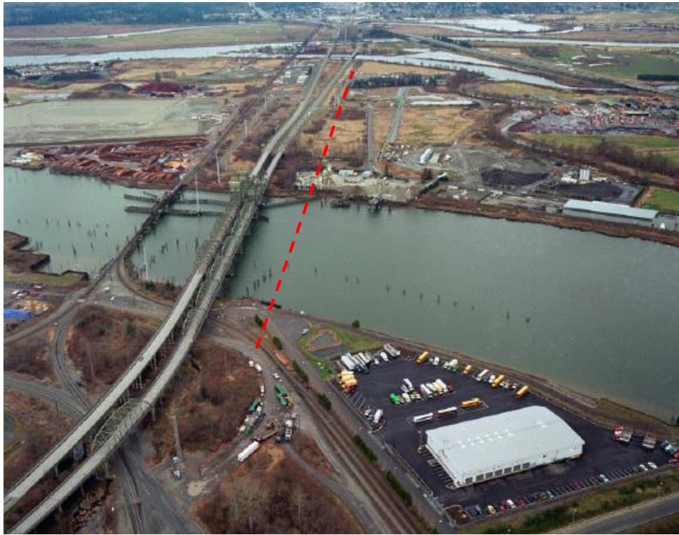
Segment 3 crossing of Snohomish River looking north
