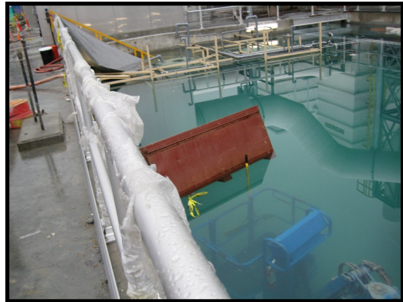
Event during construction, limited impact
