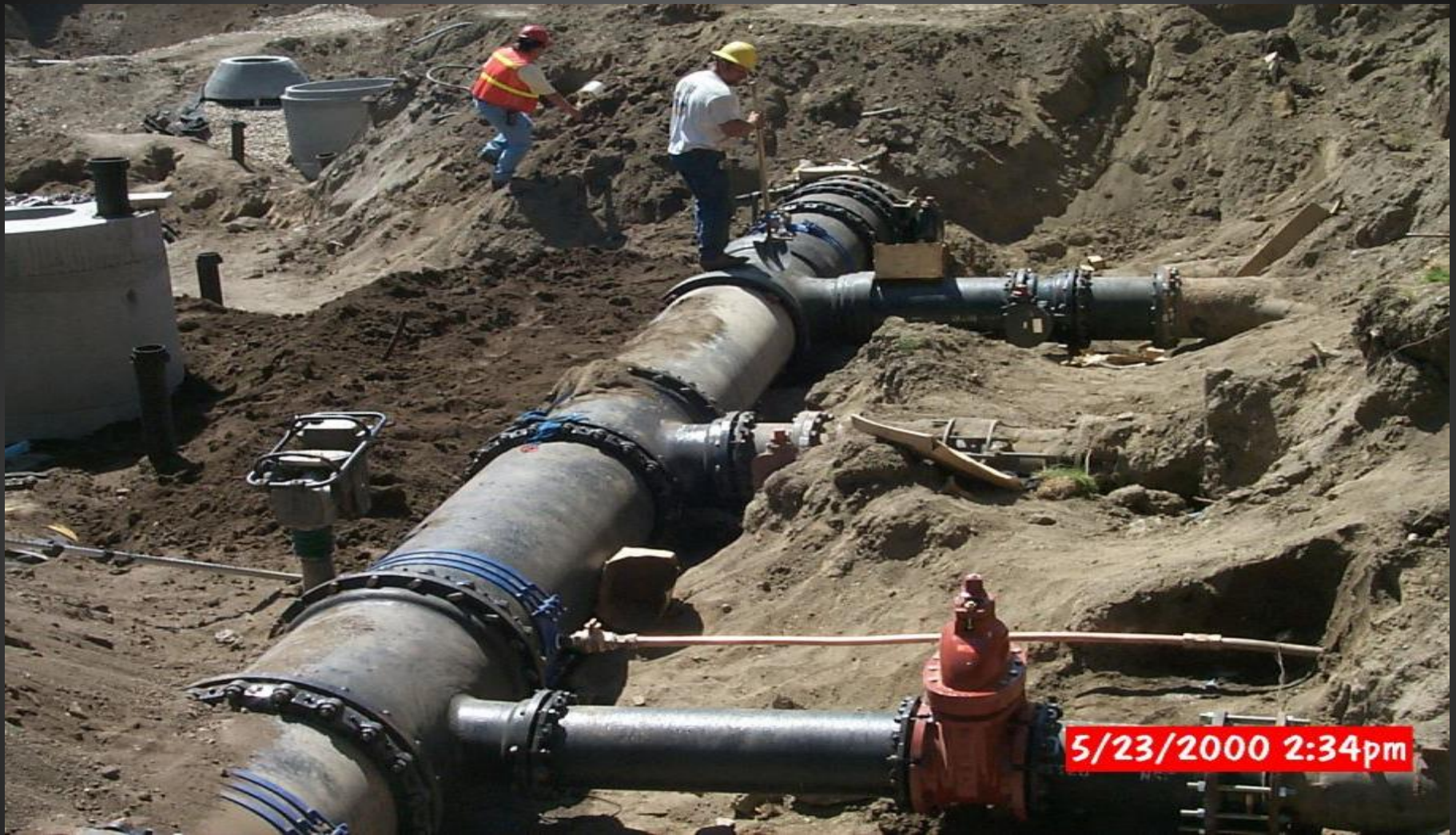
Construction of the discharge header
