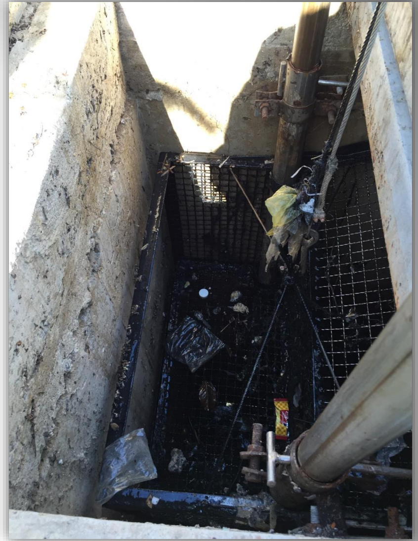
Pump station influent strainer baskets (12)
