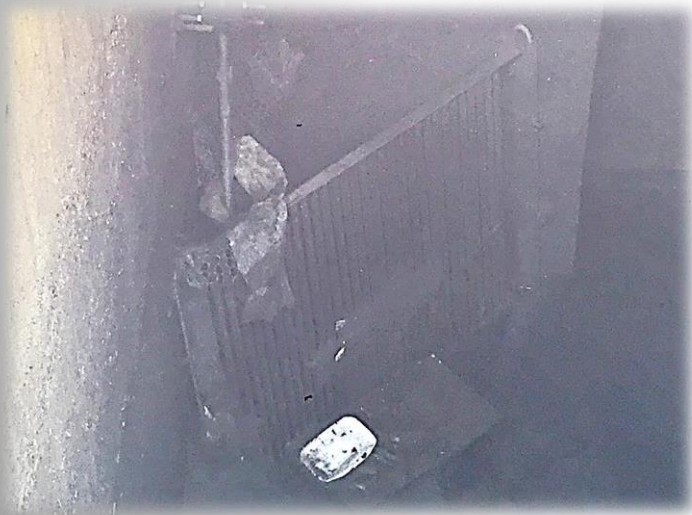
CSO Structure with Bar Screen (12)
