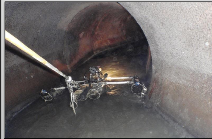
Camera in the pipe on a pontoon boat
