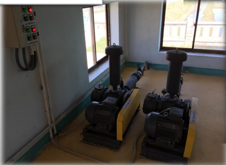
Grit Pump Air (2)
