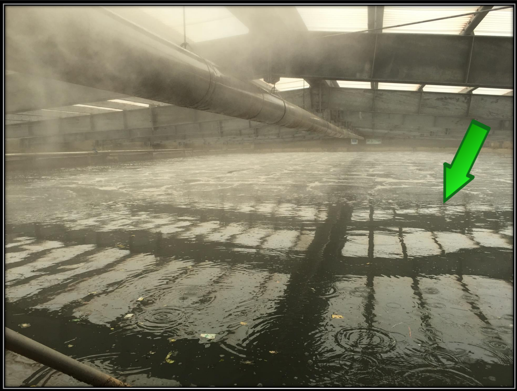
Covered Aeration Lagoon (1) note: aeration diffuser center basin only
