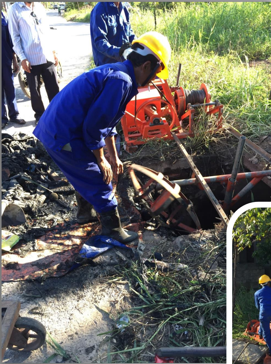
Old pipe cleaned however in unknown condition (no CCTV) Four Pipe Cleaning Machines, Six Workers/Crew (contract labor)
